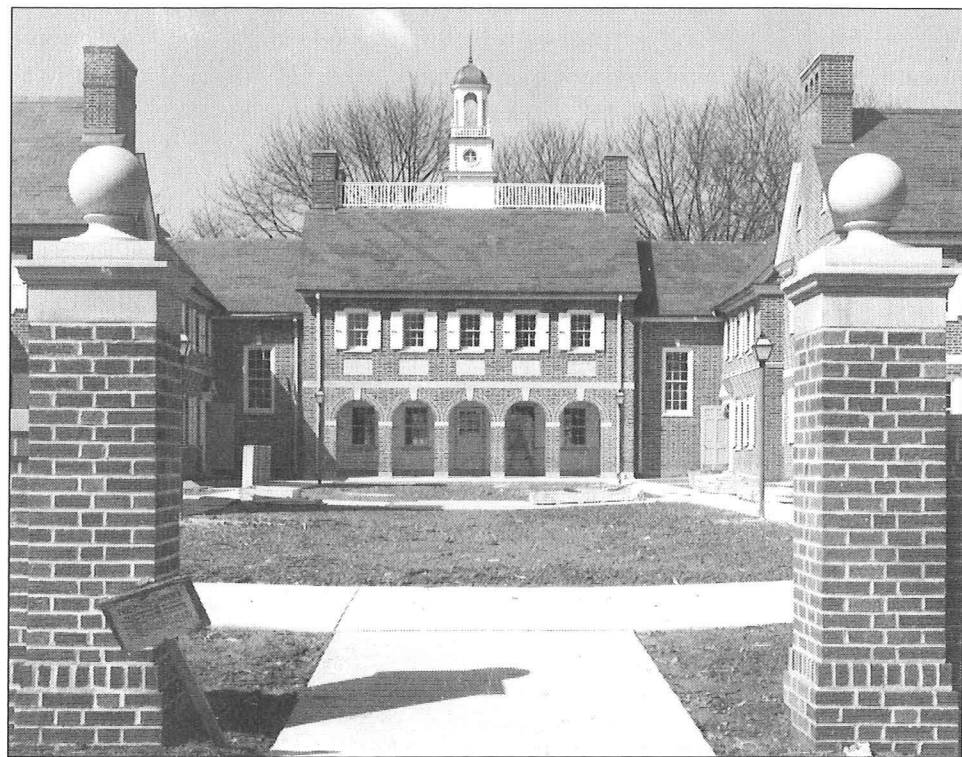
View of completed Sadler Curtilage buildings, 1952. Used with permission of the Dickinson School of Law of the Pennsylvania State University.
