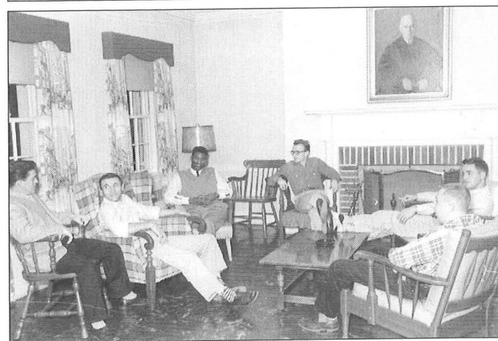
Sadler Curtilage dormitory room and common room shortly after occupancy in 1953 Used with permission of the Dickinson School of Law of the Pennsylvania State University.
