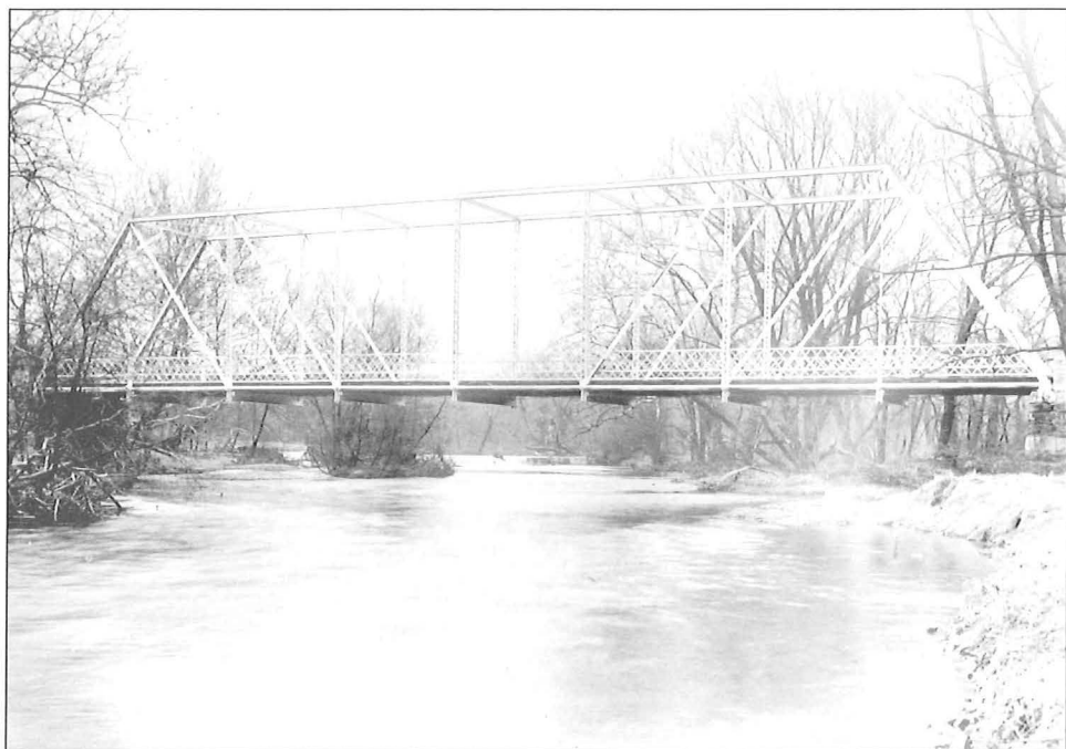
Bishops Bridge in Upper Allen Township is an iron pin truss bridge built in 1898 and still in use. 1933 photo.
