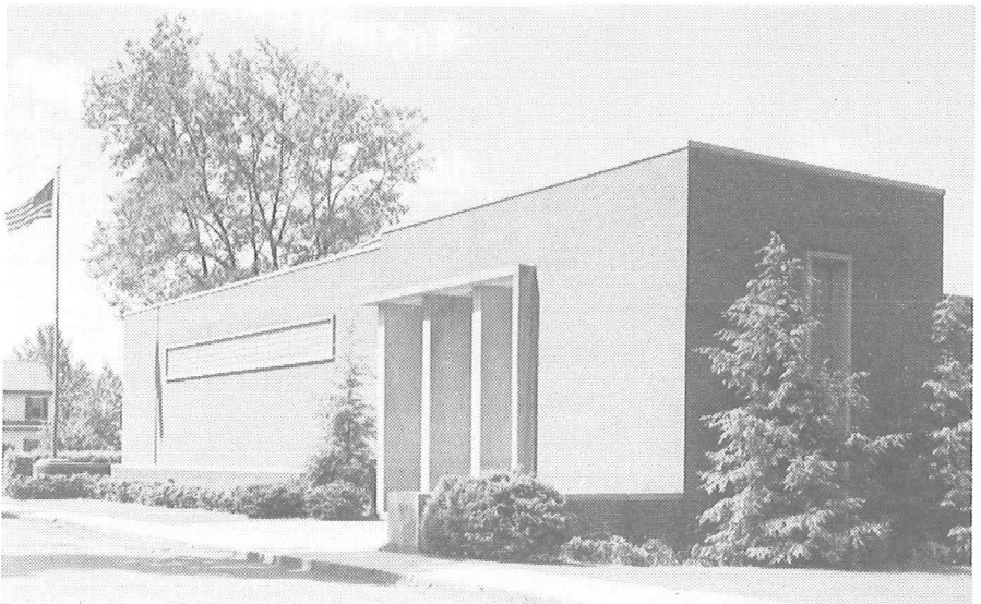
For Camp Hill School District Minick designed a high school gymnasium, auditorium, office and two classrooms on South 24th Street. The structure, erected in 1937, remains in use as part of an expanded complex to which other architects subsequently contributed. Photograph from the editor's collection.
