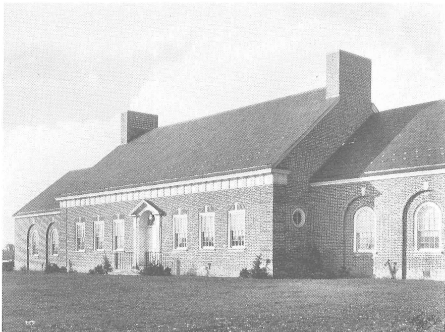
In 1929 the Camp Hill School District constructed this building, the Nathan C. Schaeffer Elementary School, after a Minick design. Note "Colonial" door, quoins, multi-paned windows, jack arches and cornice. Photograph from the editor's collection.
