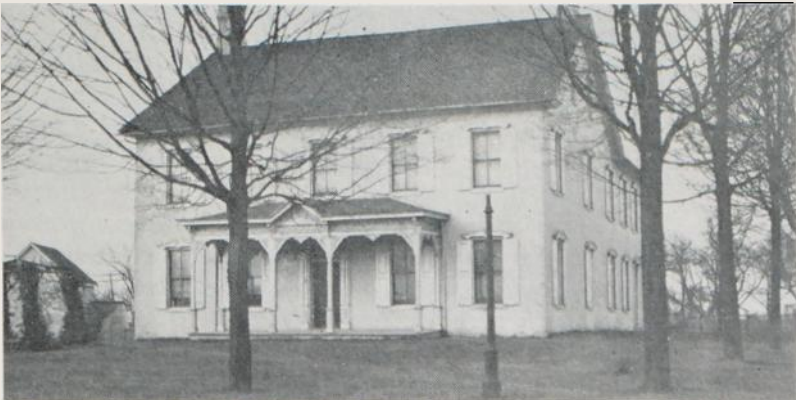
Oyster Point Tavern about 1900 when it had become a home for the Clarence Hempt family. Trindle Spring Road met Market Street at a V-shaped intersection in front of this structure.
